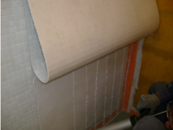
A flexible panel is handled near a wall.
