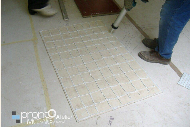
A floor assembled from prepared sections.
