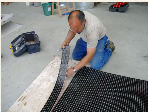
The panel is worked to the required size.
